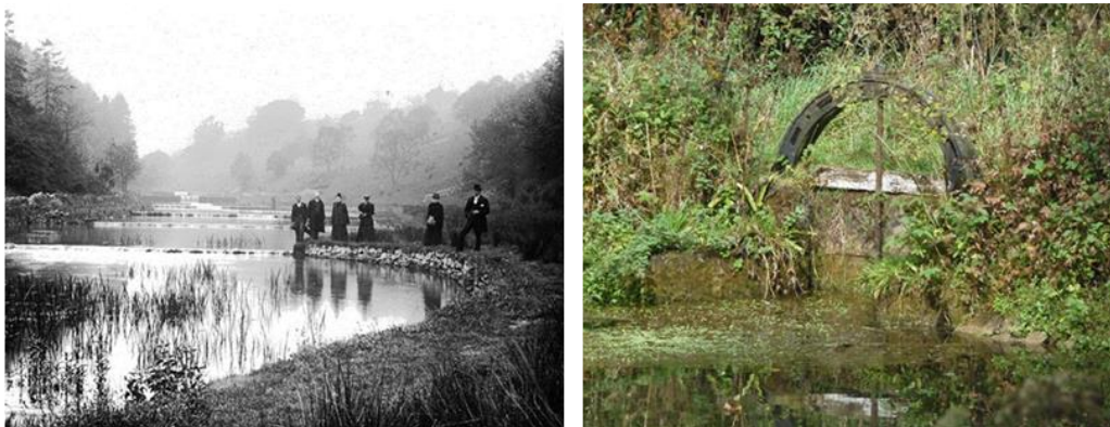
Figure 3.12 Lathkill Dale weirs (left, BHS00644, date unknown) and sluice (Photograph: Author, 2020)
