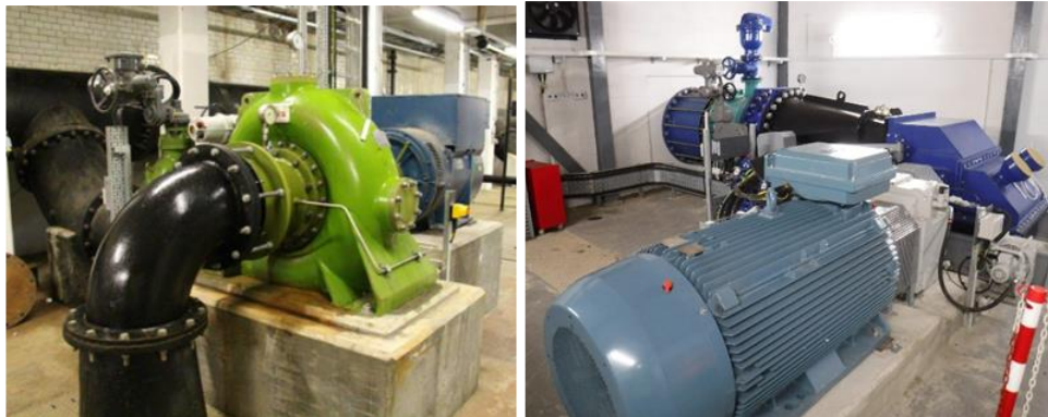
Figure 5.17 Turbines installed at Ladybower Reservoir (left) (kind permission of Ladybower Reservoir facebook) and Howden Reservoir (right) (Photograph: Author, 2019).
