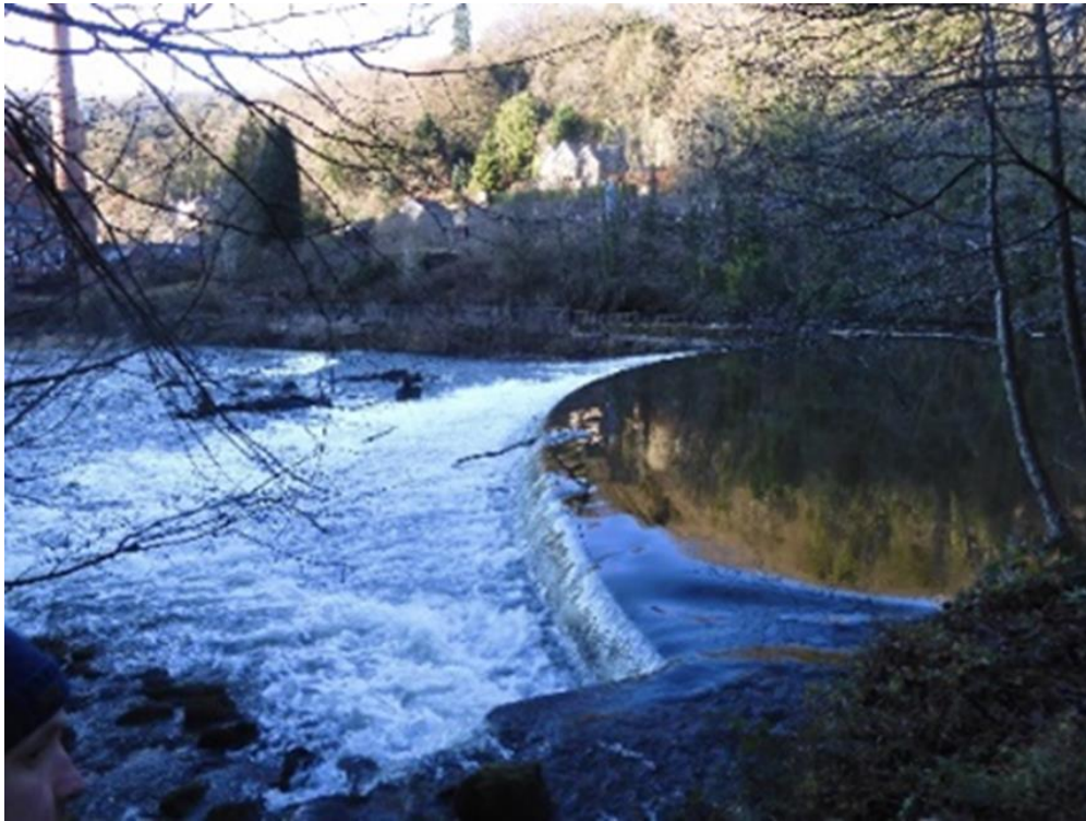
Figure 3.17 The unusually convex Masson Mills weir, possibly following a natural geological feature, a knickpoint. Photograph: Author, 2022
