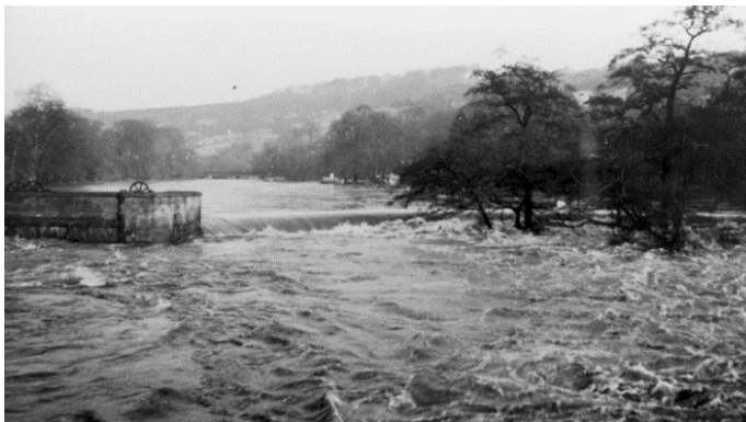
Belper: Circular weir in flood Photograph: BHS04442 (1965)
