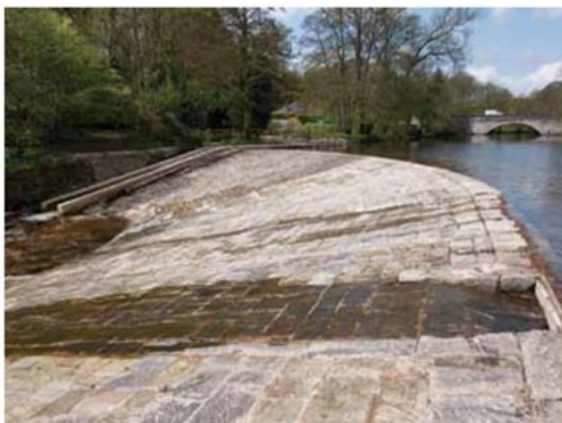
Figure 5.24 Calver weir restored 2004-2010
