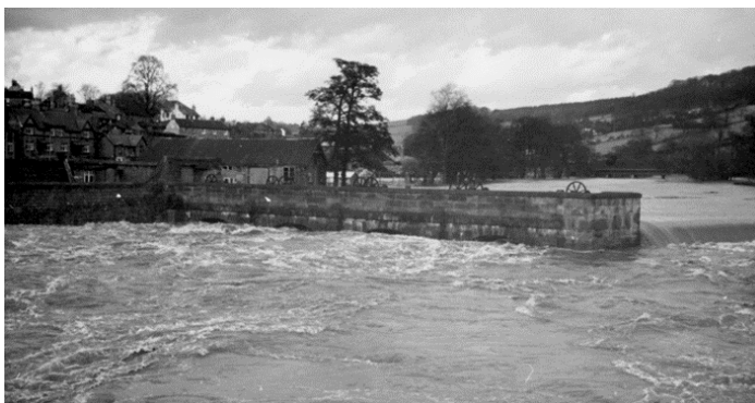
Belper: Flood-gates open in flood Photograph: BHSb1271 (1965)
