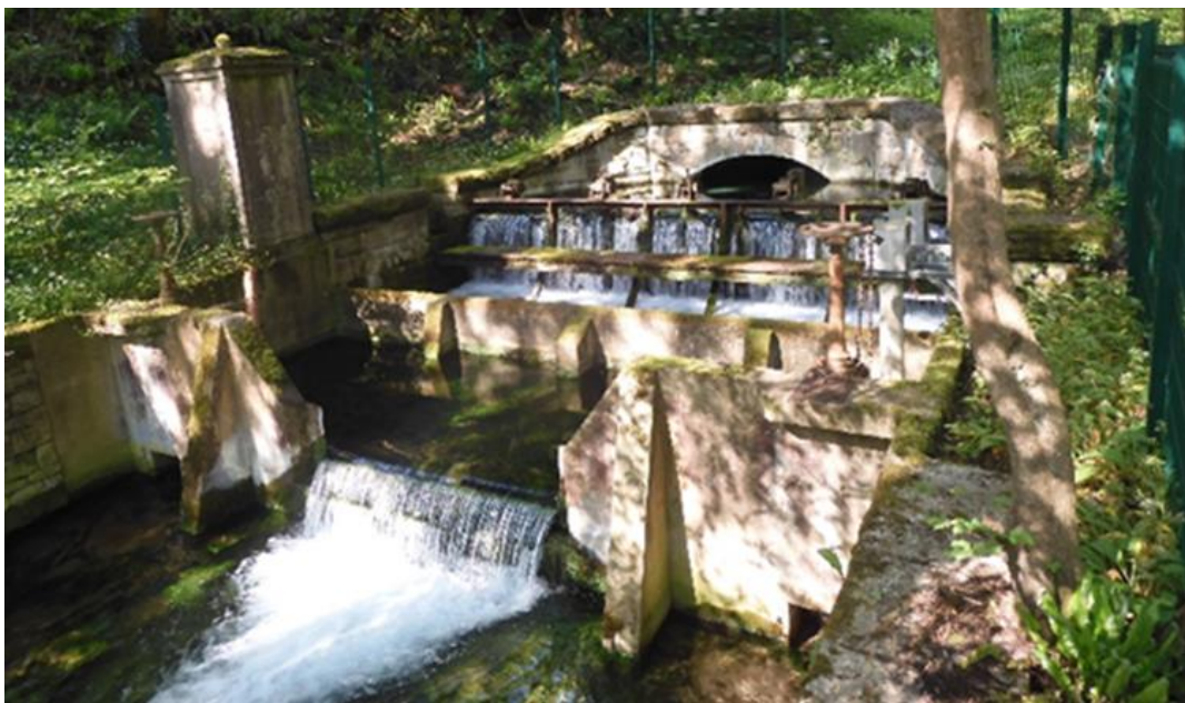
Figure 4.23 Meerbrook sough tail, main flow diverted to the right, supplying the STW Homesford water treatment works (Photograph: Author, 2021)
