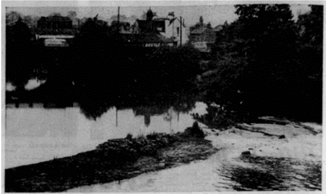
Figure 4.28 St Mary's weir Derby 1946 (Source: Historic England Archive, EAW002467) and 1968 (Derby Evening Telegraph, 1968)
