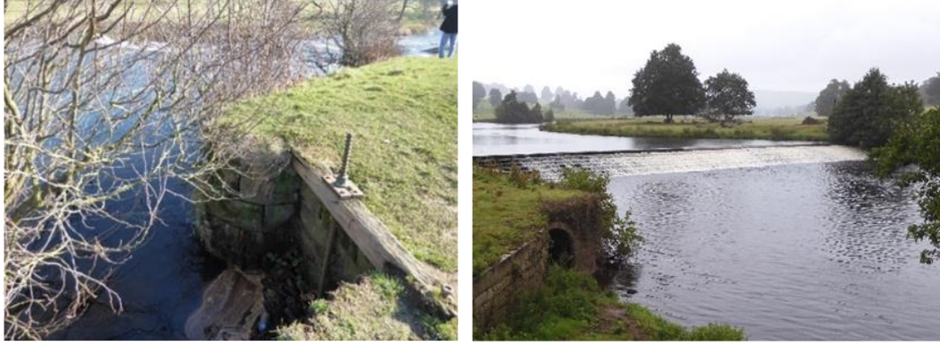
Figure 3.13 Chatsworth sluice and upper weir (Photographs: Author, 2020)
