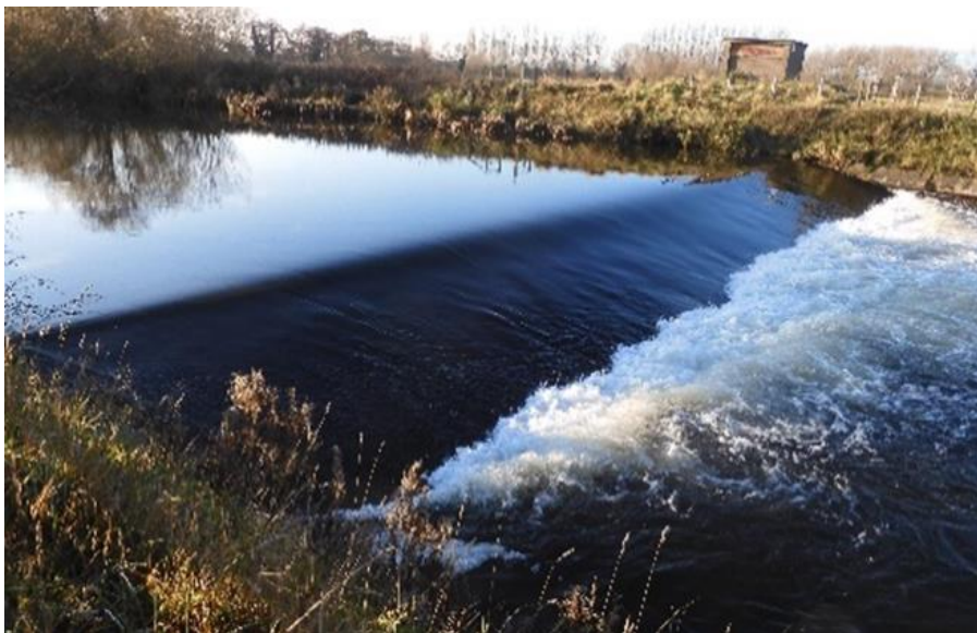
Figure 4.26 Church Wilne river gauge weir (Photograph: Author, 2022)
