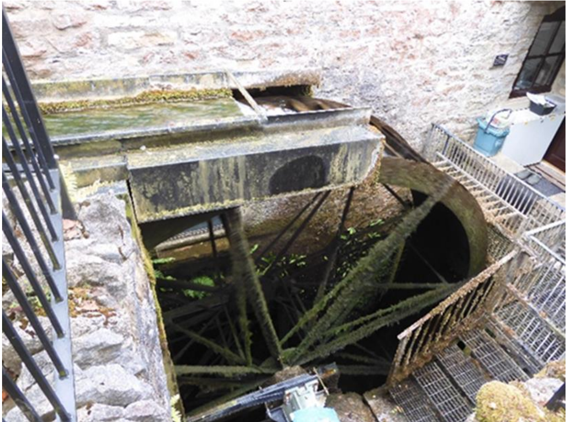
Figure 2.10 Private house (former Calver corn mill), powered by the Calver Sough, 10 kW installed in 2010 (Photograph: Author, 2021)
